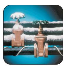
**Constant Wattage Cable** This style of heat trace cable is designed to put out a certain amount of wattage per linear foot at a particular voltage. It is always putting out the designed watts per foot, no matter what the surface or ambient temperature is. This means that in most situations the heating cable is continually pumping heat into the vessel or pipe being maintained or heat-
